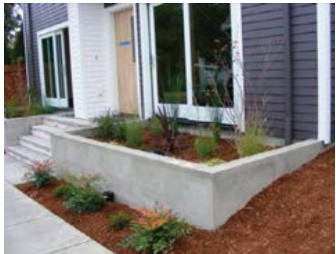
Example of a typical residential bioretention cell which holds and infiltrates stormwater on site LA TEAM EFFORT
