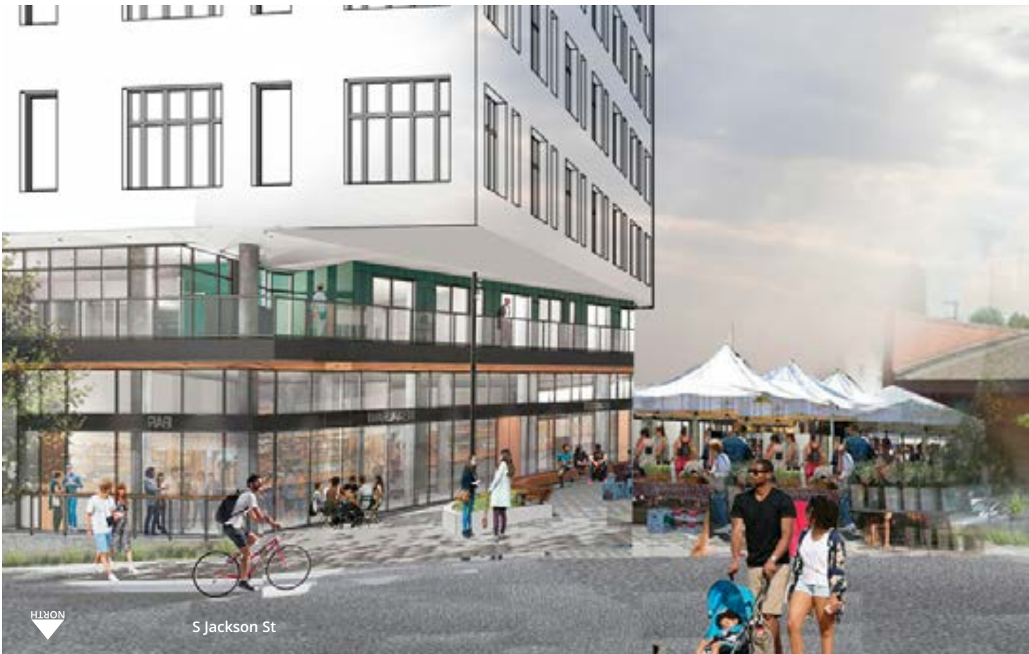
Events prompt lively interaction in the plaza between the Tabernacle sanctuary and the proposed NE corner building along S Jackson St. To the south, rowhouses and townhouses with shared greenspaces match the calmer energy of the residential neighborhood.
