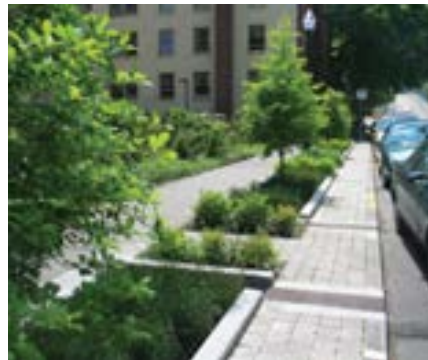
Bioswales on SW 12th Ave in Portland, OR retain and clean runoff from paved surfaces. CITY OF PORTLAND
