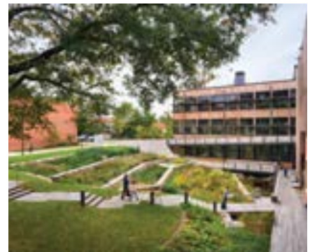
Biofiltration planters form terraced seating at Sidwell Friends School in Washington, D.C. ANDROPOGON ASSOCIATES
