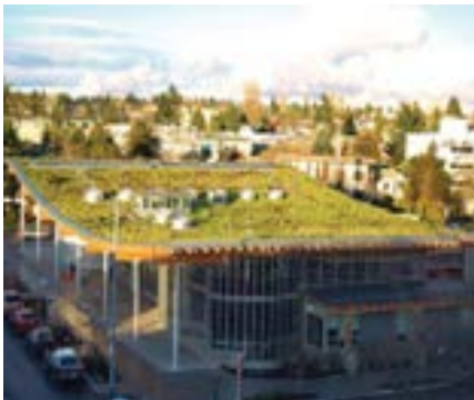
A green roof at Ballard Public Library in Seattle detains rainwater. BOHLIN CYWINSKI JACKSON
