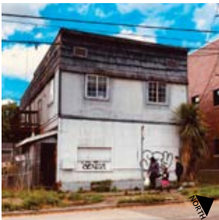
MLK site, existing structure (to be replaced)
