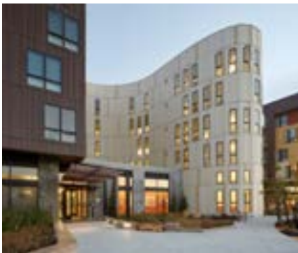
Shared courtyard, Dr. George W. Davis Senior Center, San Francisco, CA DAVID BAKER ARCHITECTS
