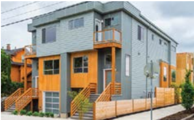
Townhouse duplexes offer efficiencies of shared-wall living combined with the increased light and outdoor space of detached housing styles. FIRENZE DEVELOPMENT, INC
