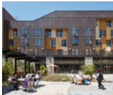
Shared courtyard, Dr. George W. Davis Senior Center, San Francisco, CA DAVID BAKER ARCHITECTS
