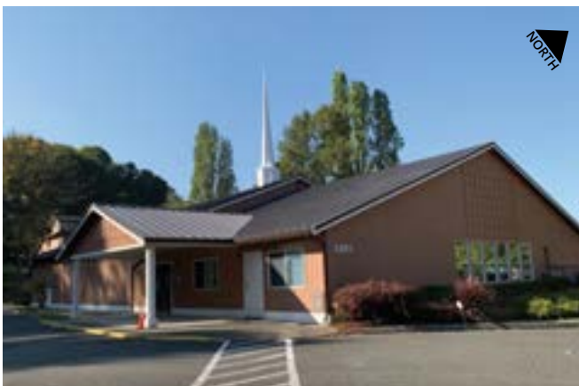
Damascus existing church building, built in 2001
