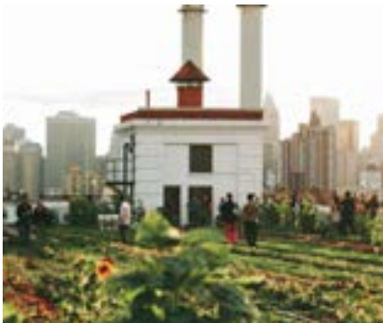
A green roof in Brooklyn, NY absorbs rainwater, grows food, and provides event space. BROOKLYN GRANGE
