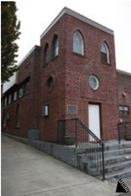
Existing Tabernacle administrative building (to be retained)
