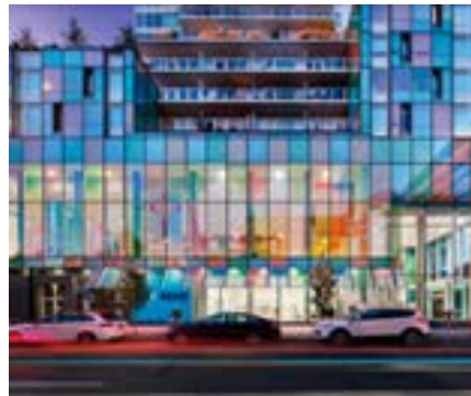
Sanctuary in new building, Central Presbyterian Church, Vancouver, BC HENRIQUEZ PARTNERS ARCHITECTS
