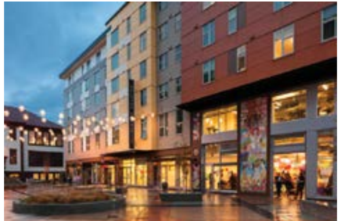
Apartments in the Central District that are human scale and encourage lively streets. CANDG
