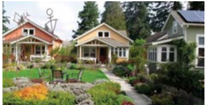
Single-story cottages clustered around shared outdoor spaces offer a neighborly and ADA accessible detached housing option. WAKE COHOUSING
